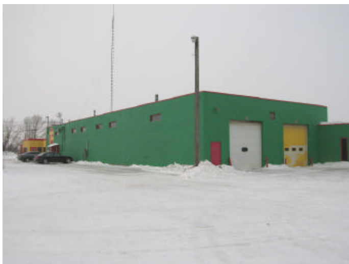
Shop/Office West View
